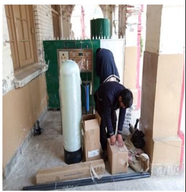
Figure 4: Installation of RO system in Govt. Shuhda-E-APS Memorial High School, Sahiwal
